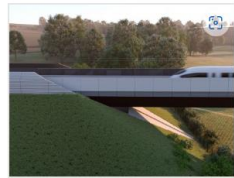
Design, Engineering and Architecture
